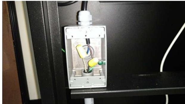
**Figure 10 - Connect Incoming AC Power per local code and NEC**
