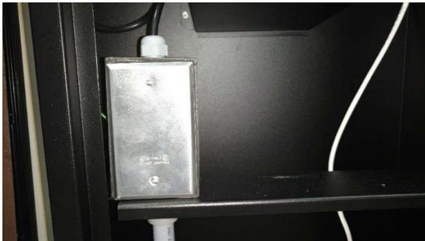
**Figure 11 - AC Connection Complete, Junction Box Sealed**
