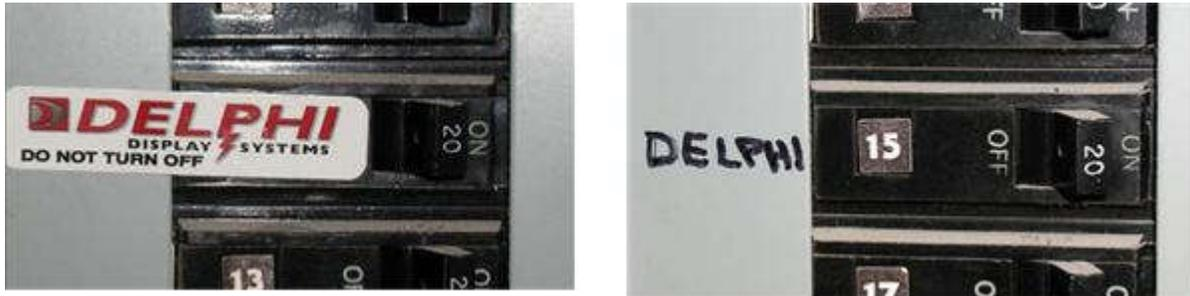
Figure 12 - Examples of Properly Labeled Circuit Breaker
