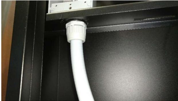
**Figure 9 - Incoming AC Electrical Routed Into Junction Box**
