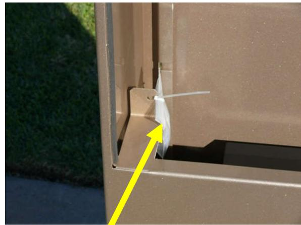
Key located inside front of Speaker Post in a plastic bag tie strapped to the mounting bracket
