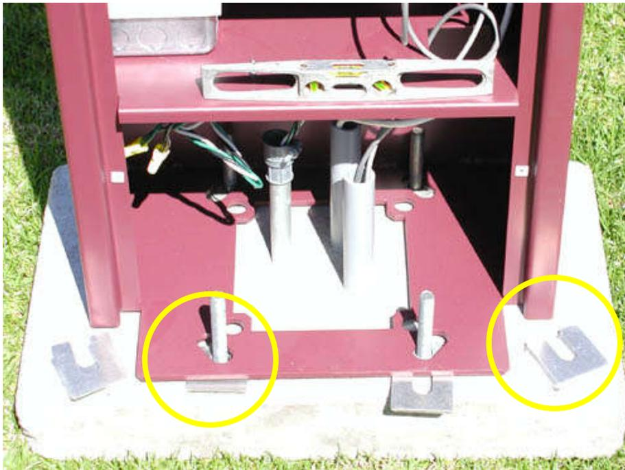
**Figure 5 - Example of Using Shims**
