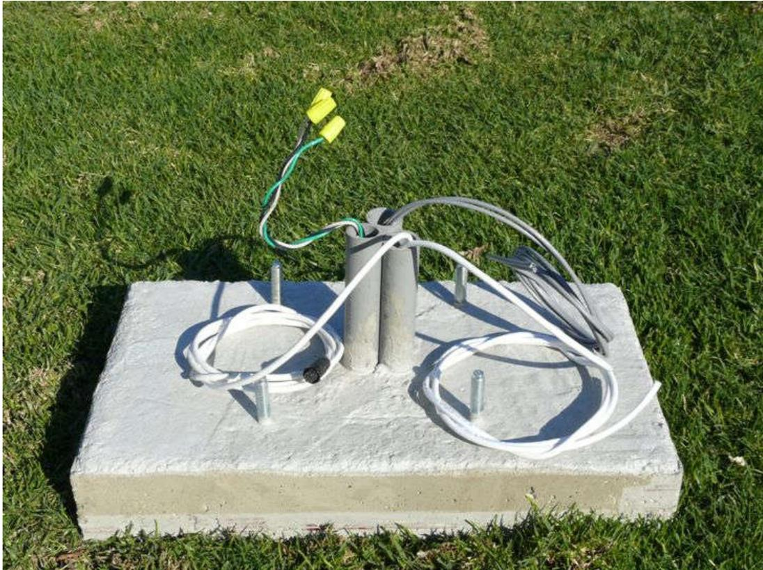
Figure 2 - Completed Footing
