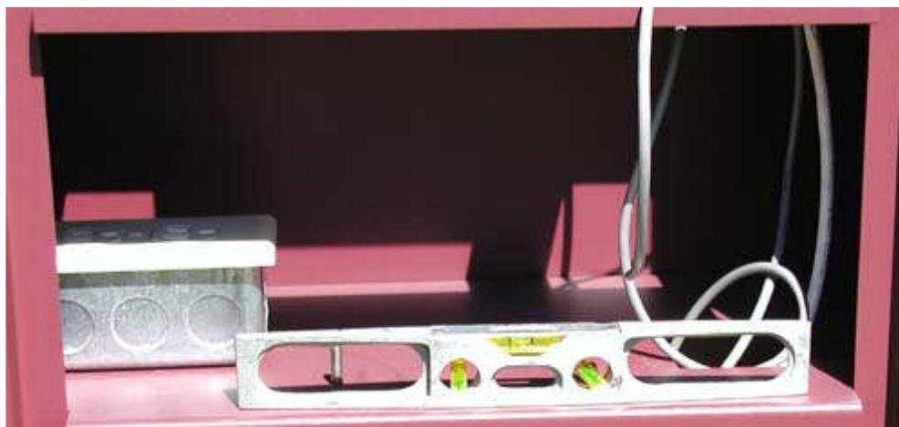
**Figure 6 - Ensure Post is Level**
